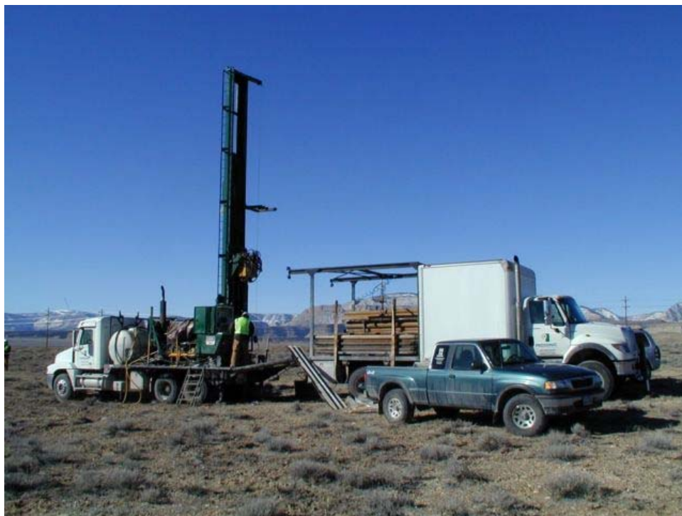
Figure D-1. Drill rig on site.
